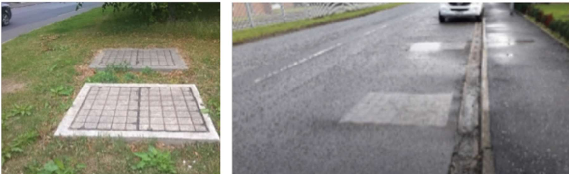
Plate 3.25 - Typical joint bays (image courtesy of Prysmian)
